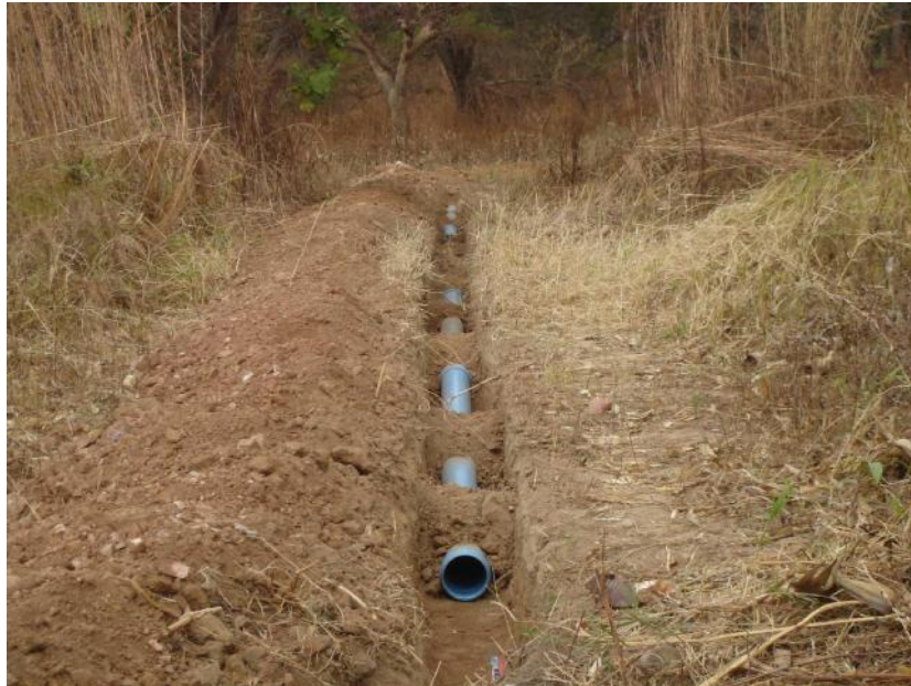
Installation of sewage plumbing during renovations.
